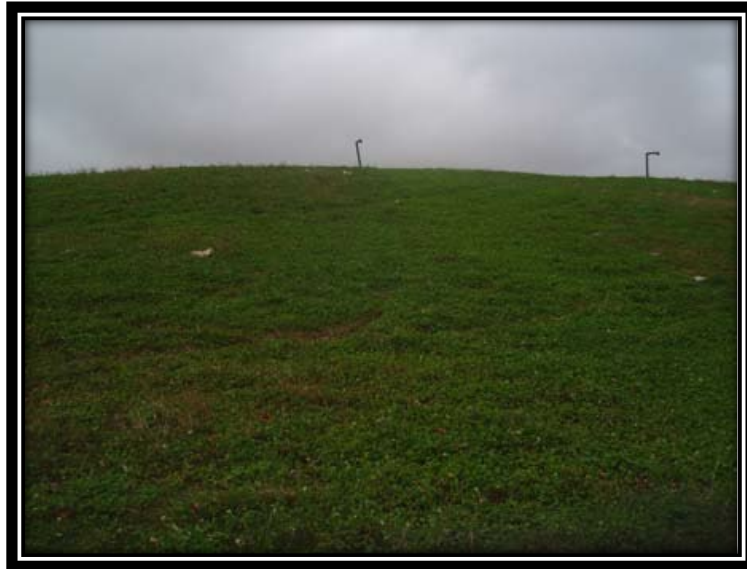
Greenville Landfill Closure
